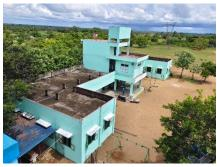
As many of you are aware, the roof of our R.C. Primary School had been damaged, leading to water leakage during the rainy season and causing difficulties for our children. To ensure a safe and conducive learning environment, essential repair work has been undertaken. This includes fixing leaks and cracks, strengthening weak areas, and repainting the school building, thereby making the structure more secure and welcoming for our students.
